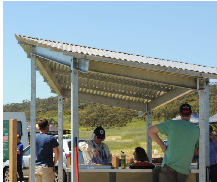
PARK SHELTERS WITH BBQ FACILITIES
