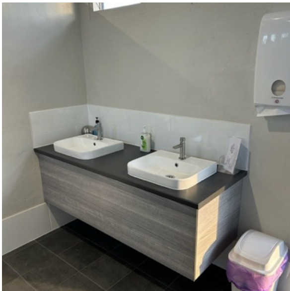
RV Park Toilets Internal Upgrade: Twin hand basin unit.
