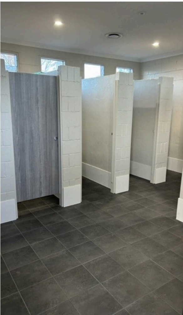
RV Park Toilets Internal Upgrade: New toilets, doors, and overall clean look.
