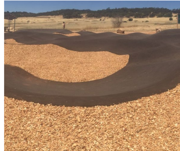
ASPHALT SEALED PUMP TRACK
