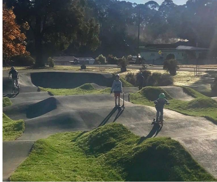
ASPHALT SEALED PUMP TRACK
