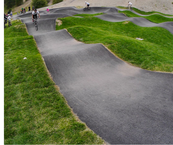
ASPHALT SEALED PUMP TRACK
